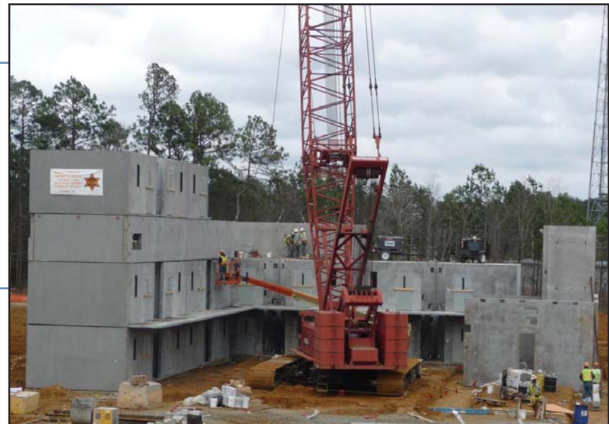
Jail Expansion - Main Wing
